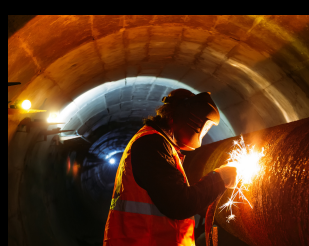
Tunnel & Subway Monitoring
